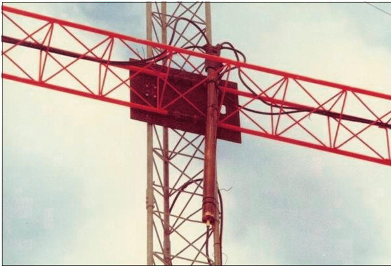
: Cross boom and power divider
