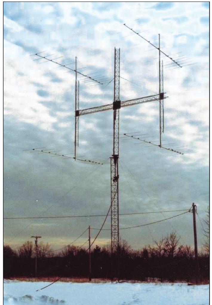
Completed array, morning after installation
